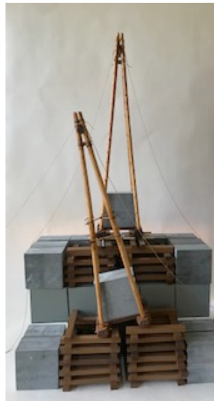
Fig. 15. A tilt levering cage on his way passing the second layer, and one standing upon the third.
